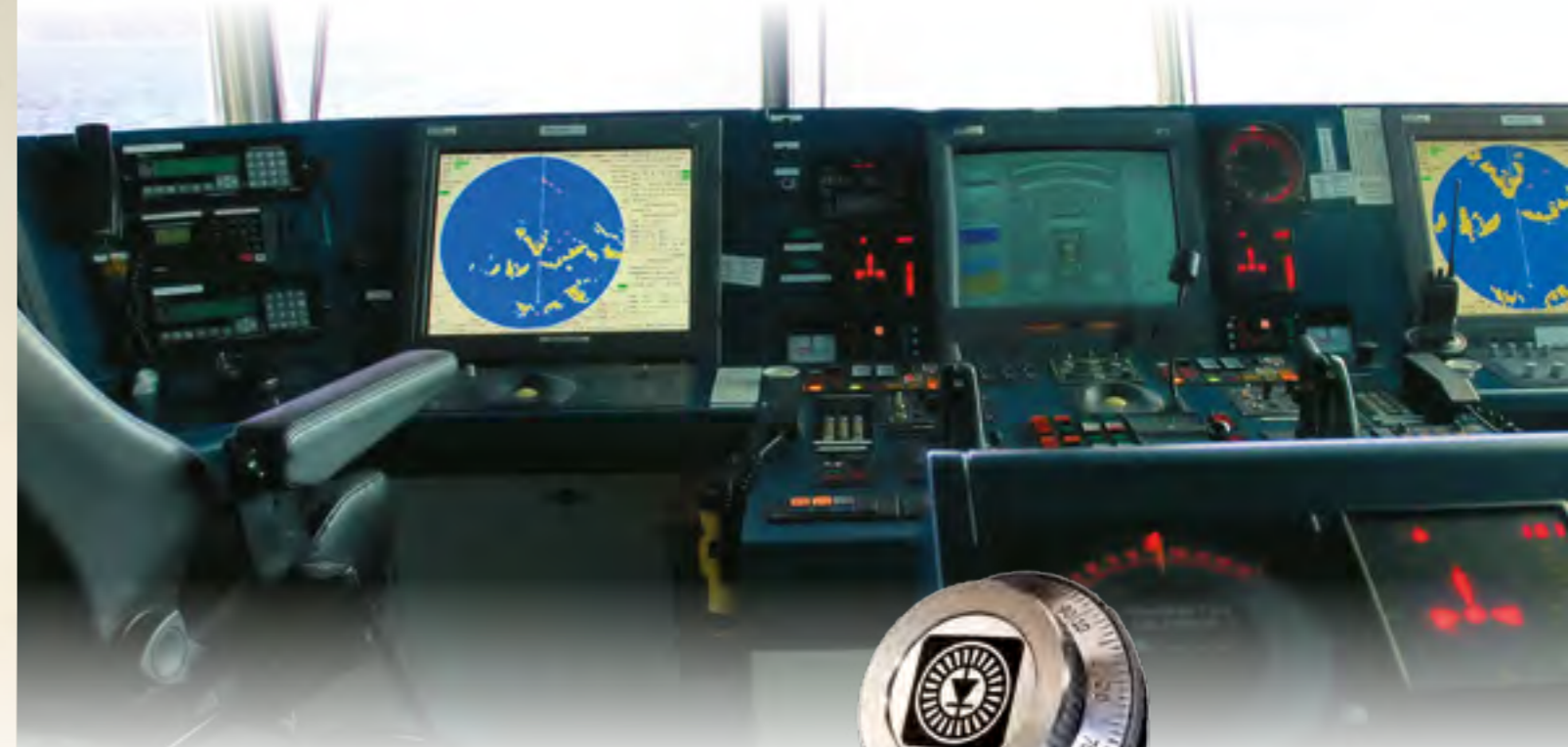
Panels on rig control house
